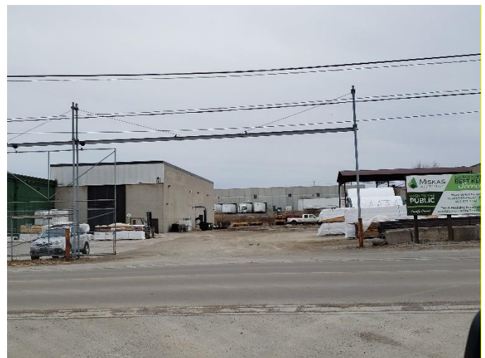
Georgetown Industrial Park
